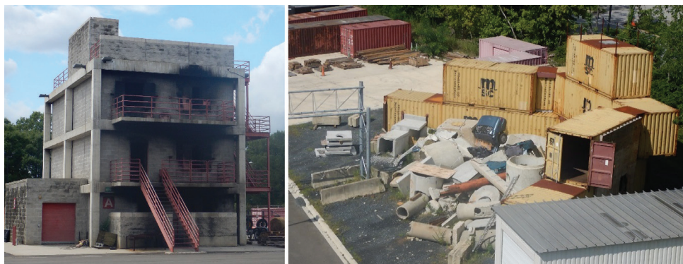
Picture 16–17: Drill building and Search and Rescue field for firefighters at the Fire Training Academy in Washington, D.C., United States
