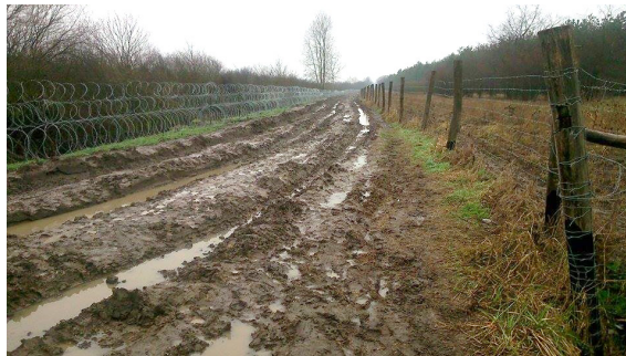
Picture 1. Manoeuvre road after a rainy day.
