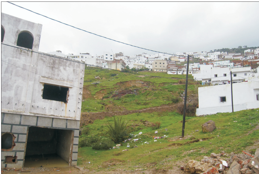
Photo 1. Consequences of landslides in Korrat Sbae before terrain management, 2012. Source: Faculty of Sciences, Tétouan, 2012.
